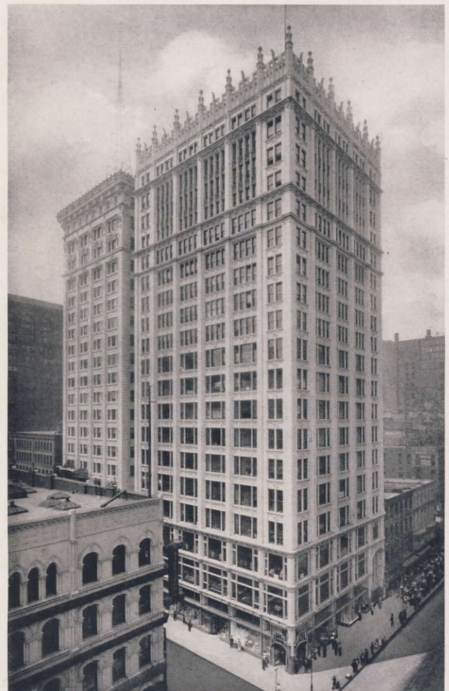
North American Bldg., State and Monroe Sts. Chicago This building reveals a striking example of the present tendency to put much architectural character at the top of the structure, to give special individuality in a city of competing sky-scrapers. Holabird & Roche, Architects. Heated with AMERICAN Radiators and Vento Heaters, installed by John R. Kehm Co. (Majestic Building at left, also heated with AMERICAN Radiators)
