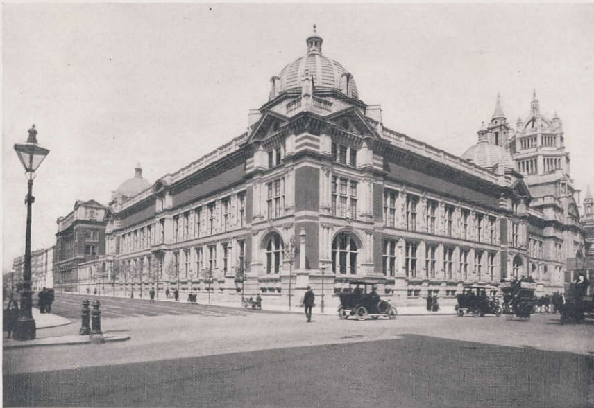
Victoria and Albert Museum, Cromwell Road, London, England Sir Aston Webb, R. A., C. B., Architect. Warmed and ventilated by AMERICAN Excelsior Indirect Radiation
