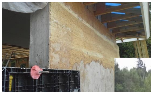
Building of the hempcrete shrine house
