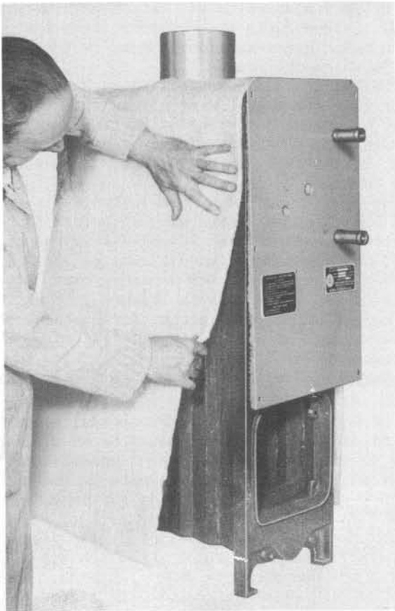
Figure 4. Installing Wrap-Around Insulation
