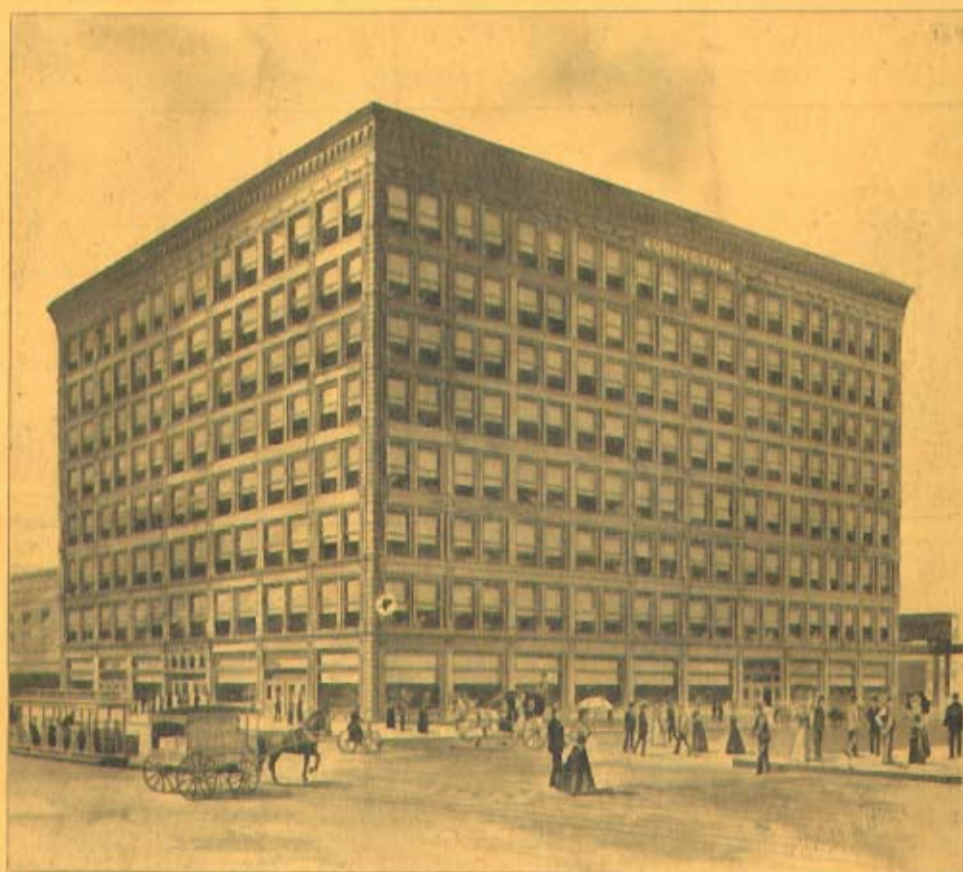
LUDINGTON BUILDING, CHICAGO.
