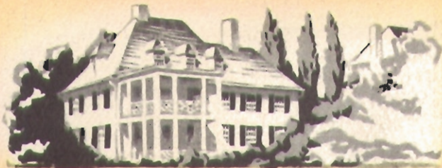
the House where the Boiler was installed
